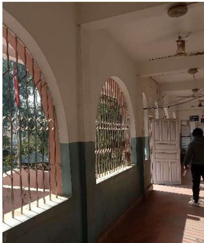
Fig: FIRST FLOOR PASSAGE
