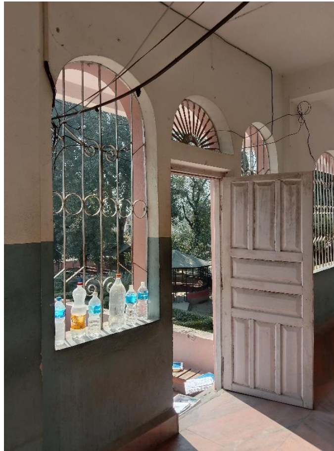
Fig: FIRST FLOOR PASSAGE
